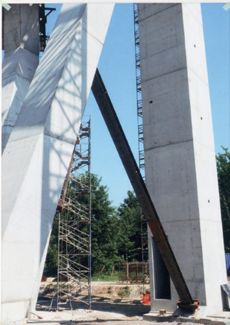
PROVISIONAL SUPPORT OF THE 'I' ON THE STAIRCASE
