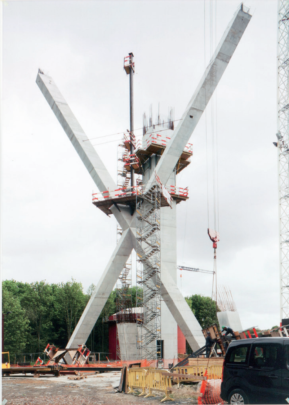
INSTALLATION OF THE CENTRAL SUPPORT BRACE. PHOTO: M. DELVAUX
