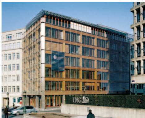
Fig. 15 | 01-489 | Office refurbishment | Marnixlaan | Brussels | 2004-2009
